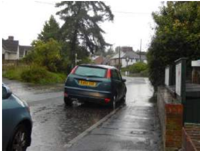
Ponding outside the village shop during the rain. 19.8.17
