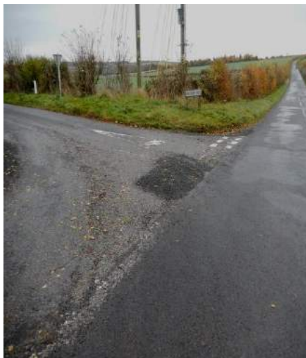
The junction at the top of Barrow Hill
