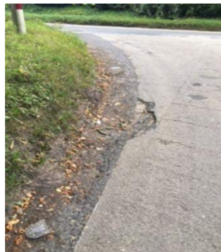
Junction of Church Lane with the A 3057
